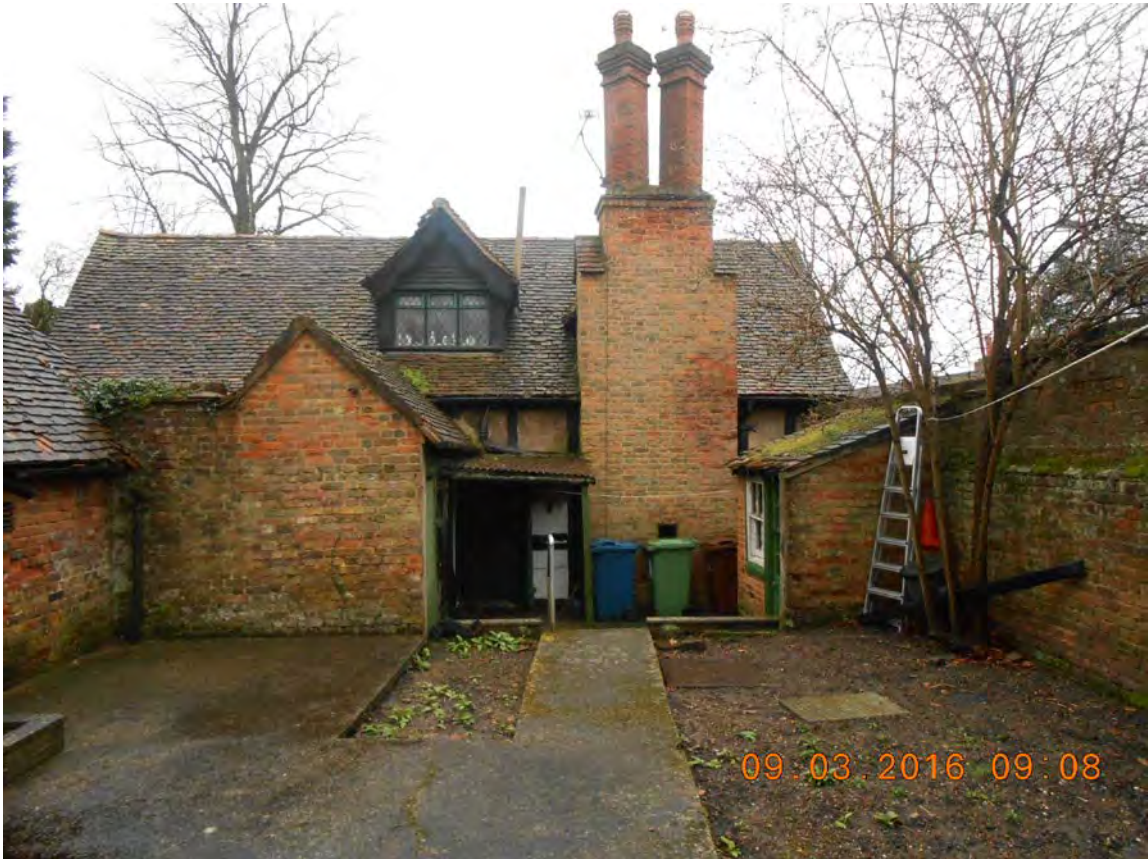
FLANK ELEVATION OF COTTAGE FROM RAISED PATIO
