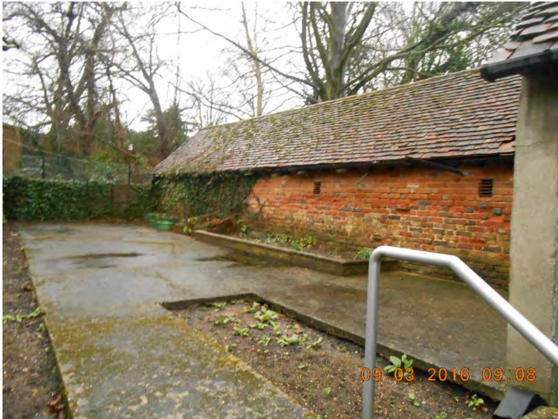
EXISTING COWSHED VIEWED FROM WITHIN PATIO AREA
